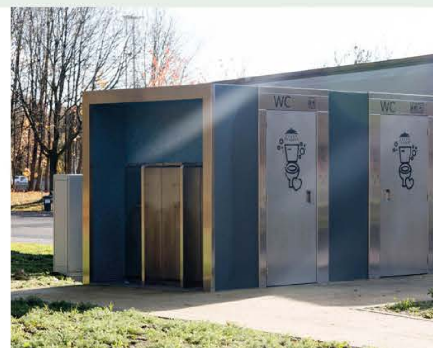
Sanitaire unit (Ilawa Forest - Landscape Architecture Lab)
